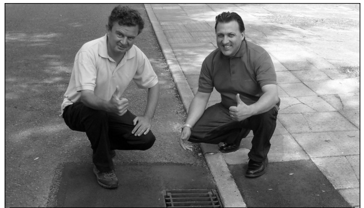
Repairs to the drains like this one in Germander Place , Conniburrow , have been actioned after requests from local residents” says Rex Exon .
