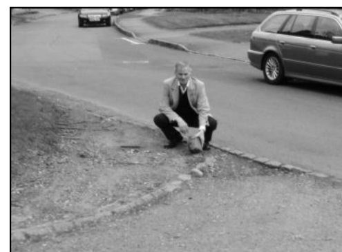
Cllr Richards, pictured right, at the bellmouth of Pritchard Court. The damage to this stone work was caused by Council Recycling lorries turning in or out of the main entrance.
