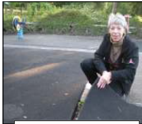
Lib Dem Vanessa McPake inspecting the dangerous play area surface.
